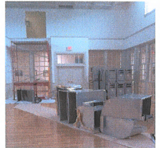
Old HVAC units being removed through the ballroom
